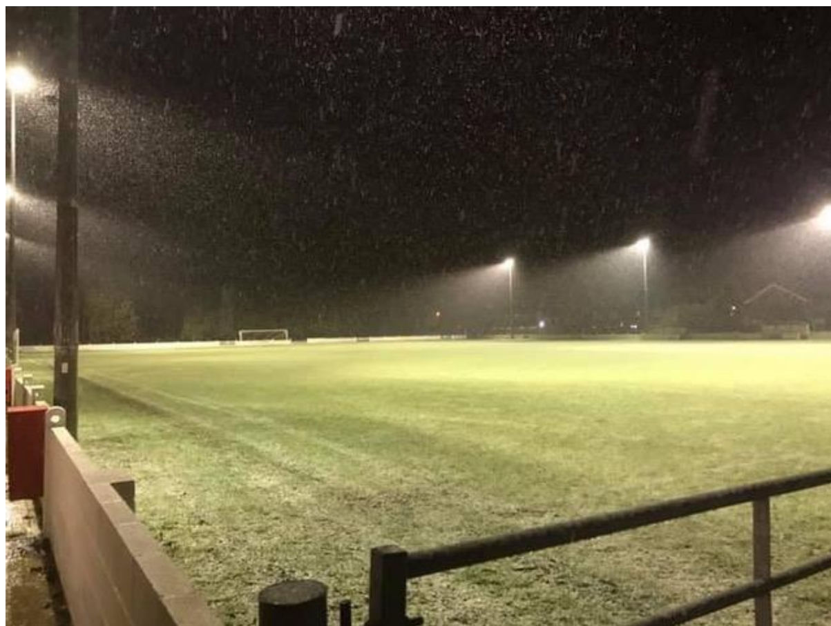
Upgraded floodlights on the stadium football pitch
